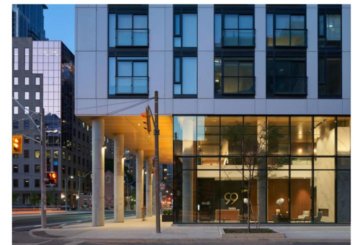
This clever approach to densification was realised by adding a new 32-storey residential tower to the existing 24-storey residential tower, and by connecting a further four levels of new residential and amenity space above the existing tower. This was achieved while ensuring the ongoing occupancy of the existing commercial and residential buildings, in addition to navigating the complexities of the urban context.
